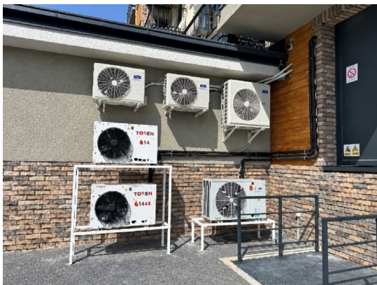
Fig. 1 Noise sources on the facade
